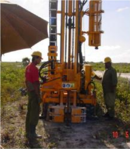
Perforadora ROLATEC RL 48L (Trabajando)
